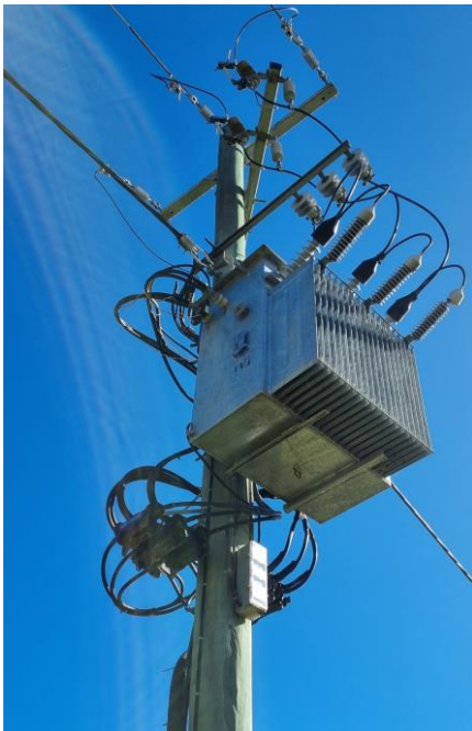
Figure 2 22kV/400/230V Pole mounted substation
