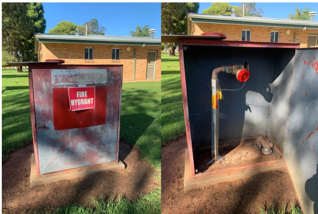
Figure 6 Existing single pillar fire hydrant the differs from the dual pillar fire hydrant specified in the fire hydrant block plan
