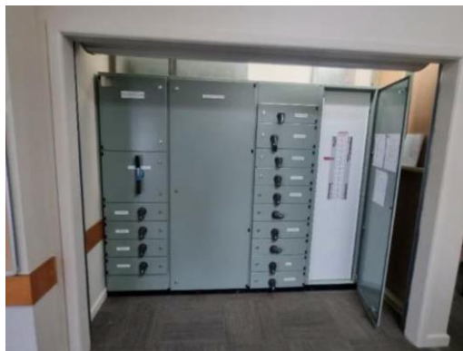
Figure 4 Existing main distribution switchboard (MDSB) Standby Power System
